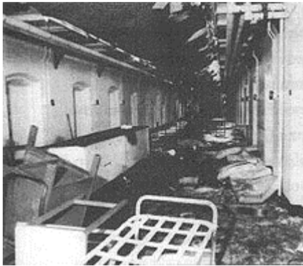
Damage caused to B wing of the prison
